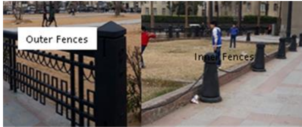
Figure 28 Outer and inner fences_Source (1)
