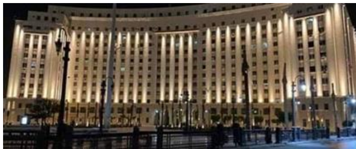
Figure 30 Some lighting poles in El-Tahrir Complex Plaza _Source (1)
