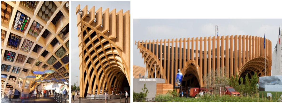
Figure 14. A structural canopy was demonstrated by WEsarch Lab using the programs Grasshopper and Rhinoceros.
